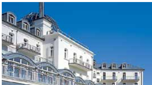
Ornamental profiles confer identity and character on a building.
