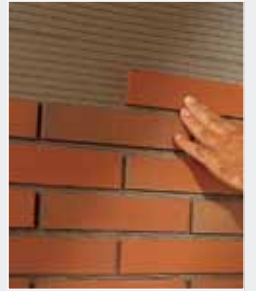
Installation using the combing method
