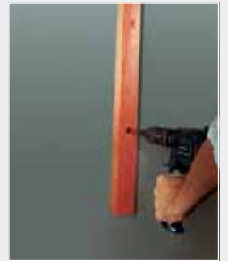
Fixing battens to the insulation
