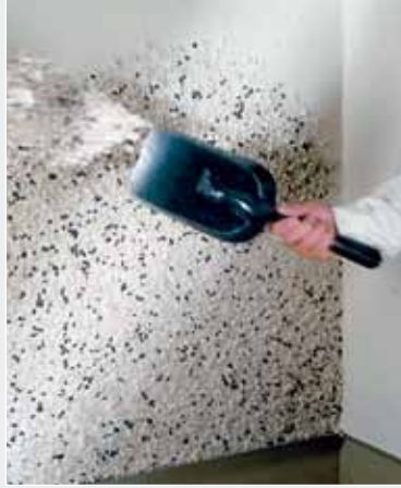
Covering the walls with Spar Dash
