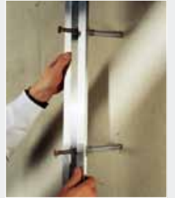
Fitting the base support with spacer plugs
